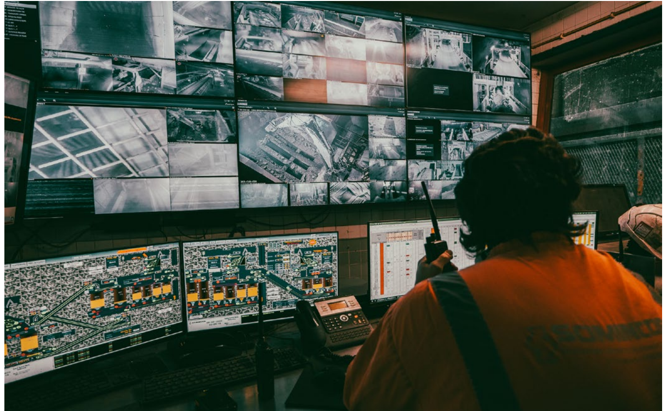
Control room, Neves-Corvo, Portugal
