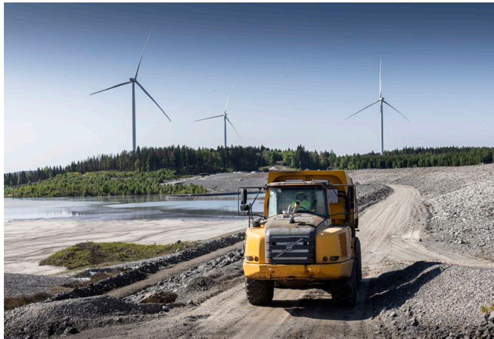
Tailings Facility, Zinkgruvan, Sweden
