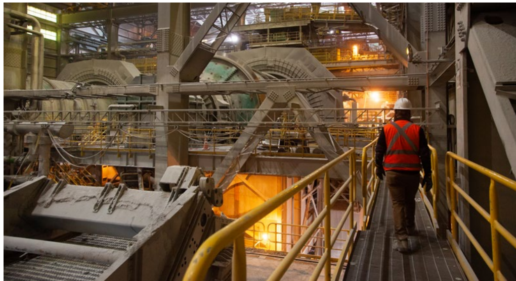
Process Plant, Caserones, Chile
