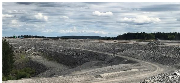
Enemossen tailings facility at Zinkgruvan, Sweden
