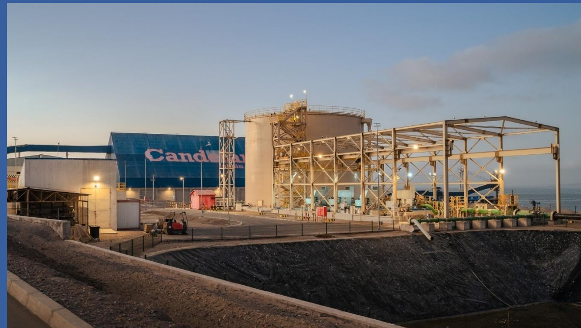
Candelaria, Punta Padrones Port & Desalination Plant, Chile
