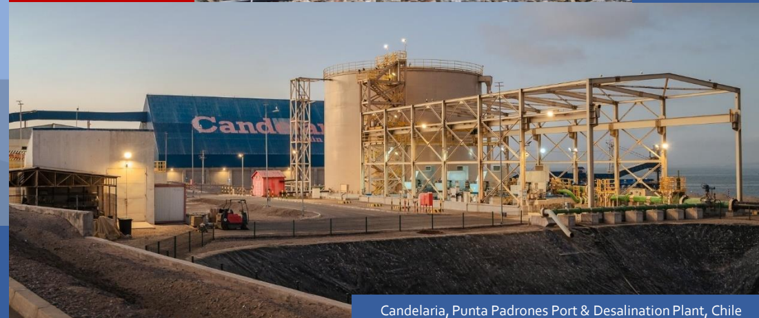
Candelaria, Punta Padrones Port & Desalination Plant, Chile
