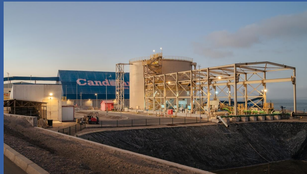
Candelaria, Punta Padrones Port & Desalination Plant, Chile
