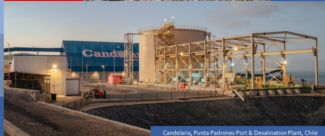
Candelaria, Punta Padrones Port & Desalination Plant, Chile
