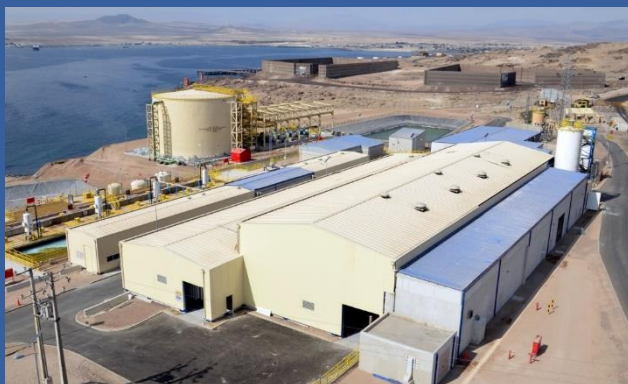
Candelaria desalination facility
