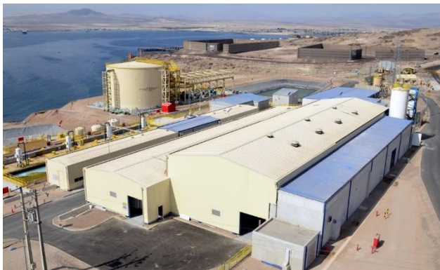
Candelaria desalination facility
