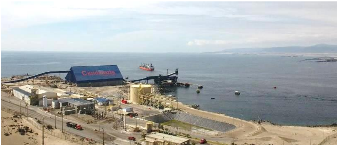
Candelaria Punta Padrones port and desalination plant
