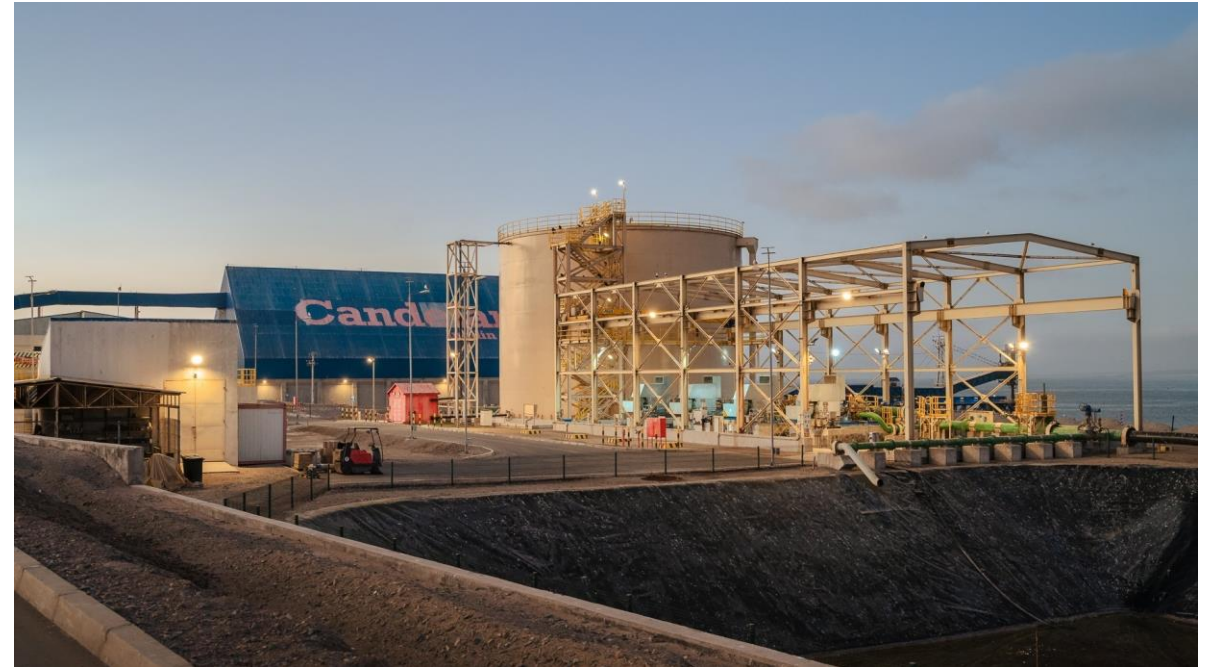
Candelaria, Punta Padrones Port & Desalination Plant, Chile
