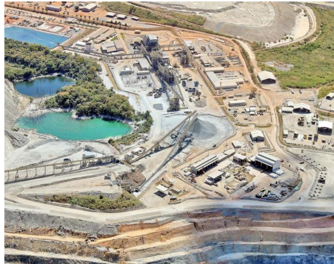
Chapada Processing Plant, Brazil
