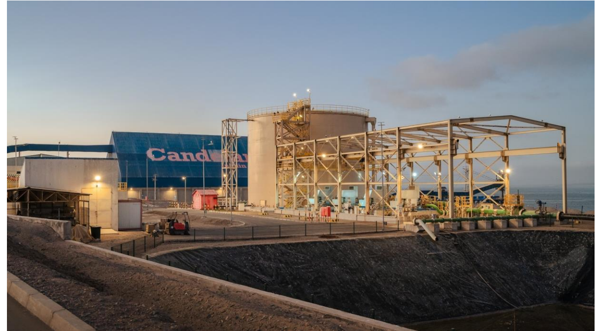
Candelaria, Punta Padrones Port & Desalination Plant, Chile
