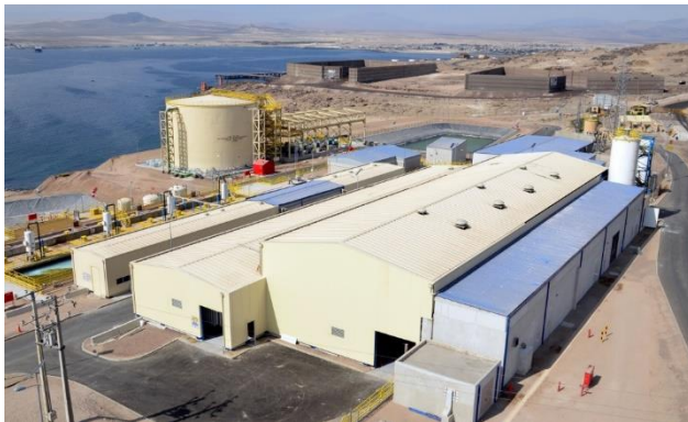
Candelaria desalination facility
