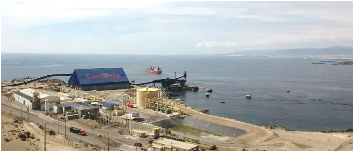
Candelaria Punta Padrones port and desalination plant
