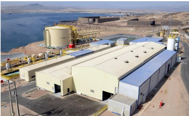
Candelaria desalination facility
