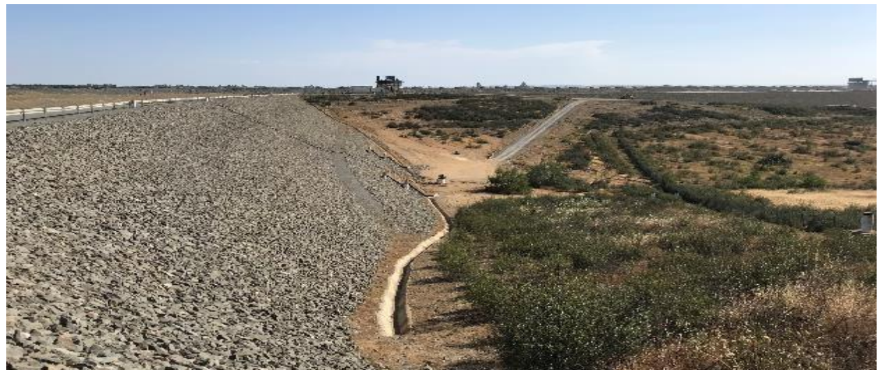
Cerro do Lobo Tailings Facility at Neves-Corvo in Portugal
