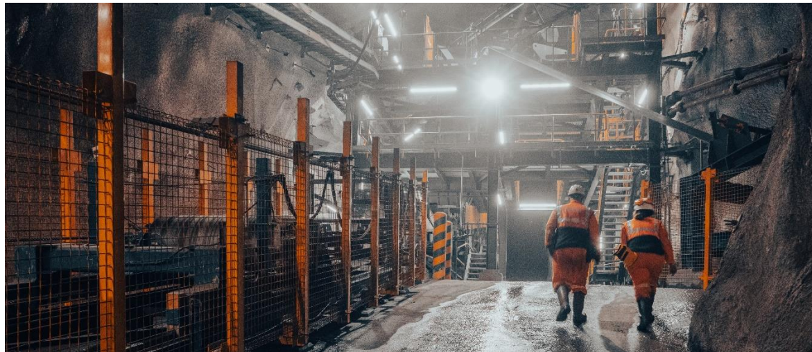
Neves-Corvo – new ZEP underground conveyor transfer tower - July 2022
