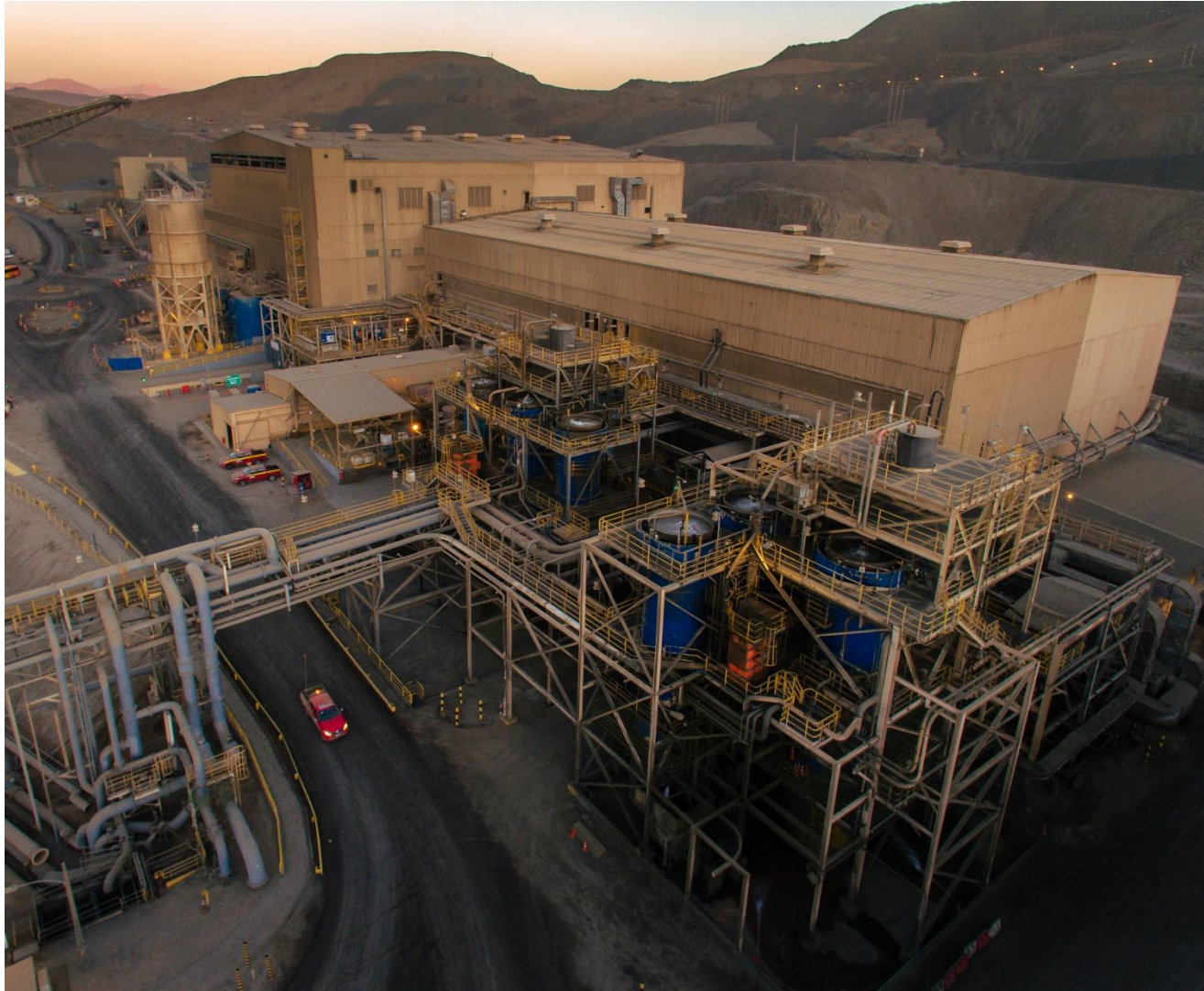
Candelaria Processing Plant – June 2022
