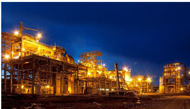
Chapada processing plant
