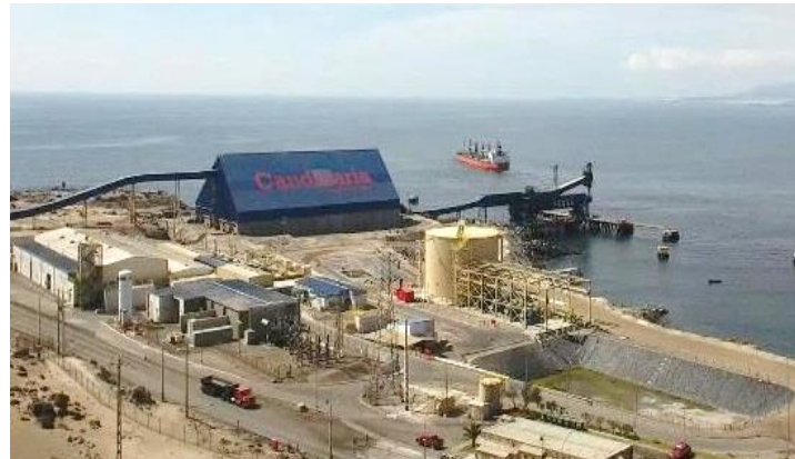
Candelaria Punta Padrones port and desalination plant
