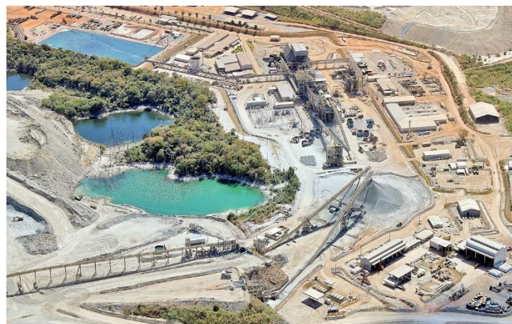
Chapada Processing Plant
