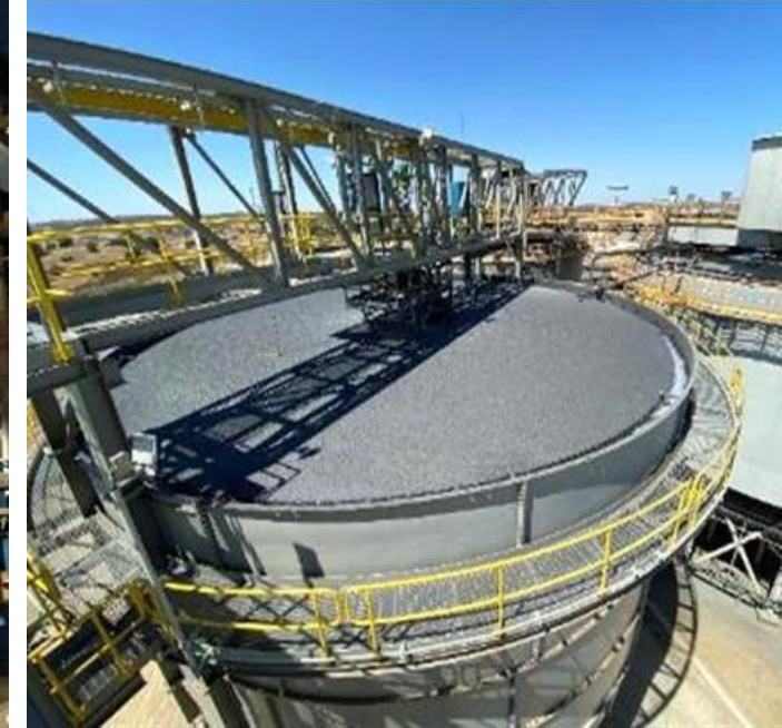
3 rd tailings paste thickener commissioned
