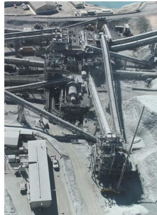
Candelaria plant pebble crushing circuit
