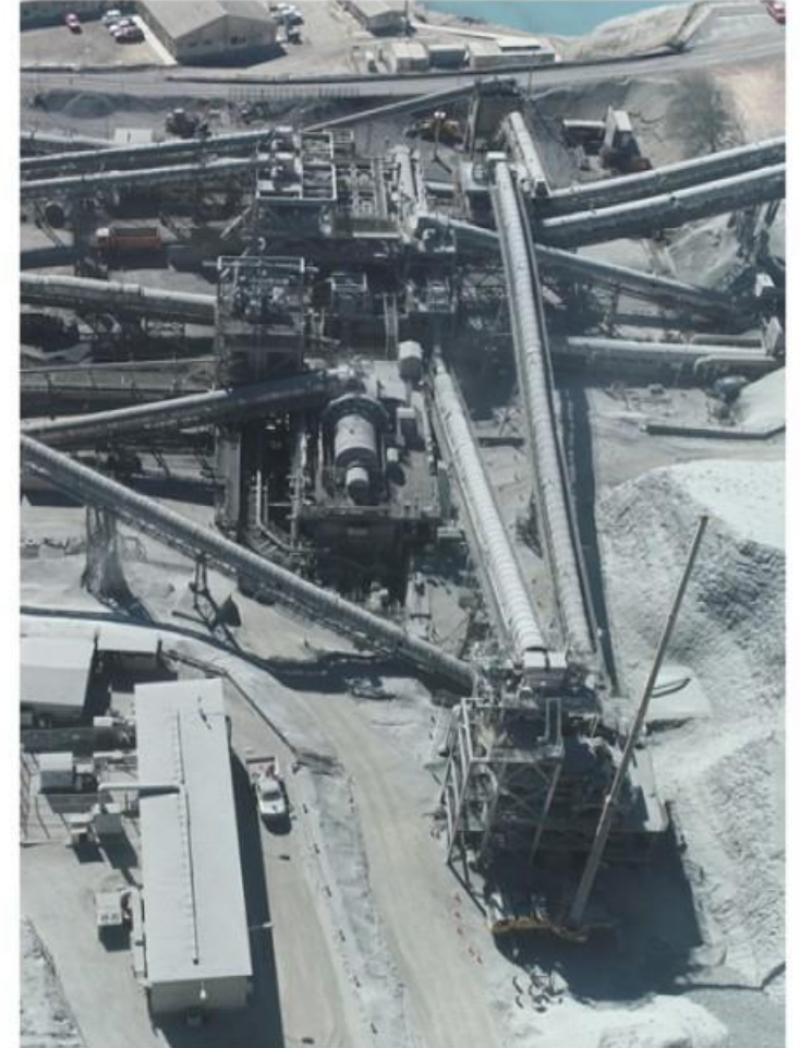
Candelaria plant pebble crushing circuit
