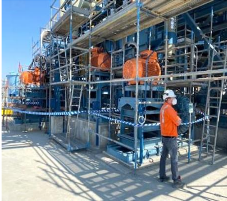
Cyclone energization and cold commissioning
