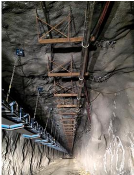
Belt and pipe support installation work completed
