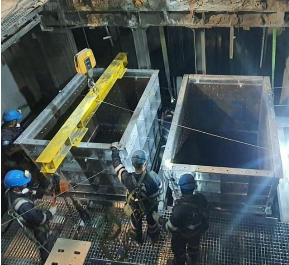
Neves-Corvo ZEP shaft upgrade work – August 2021
