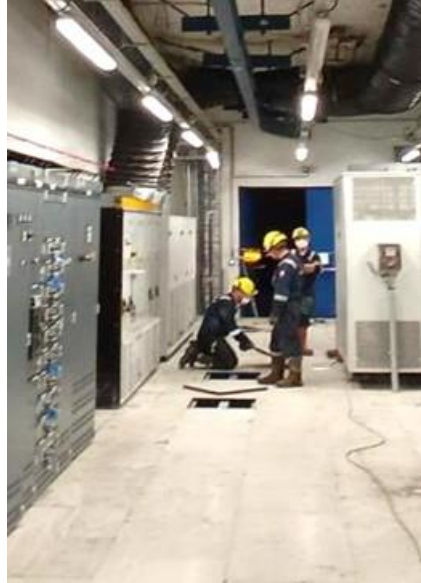
Fire suppression installation in electrical control room
