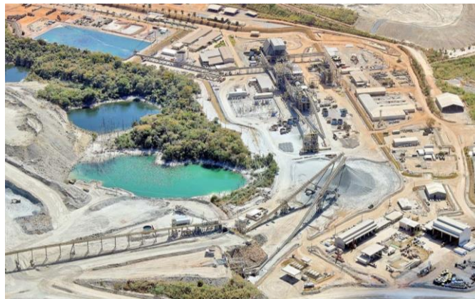
Chapada Processing Plant
