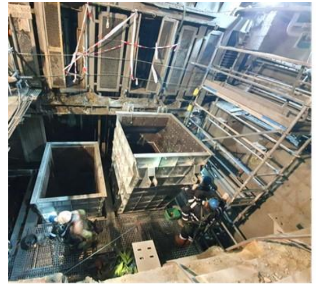
Shaft upgrade construction
