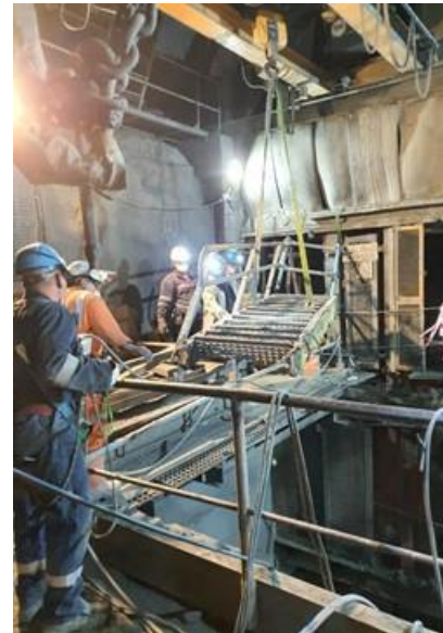
Shaft upgrade mechanical works
