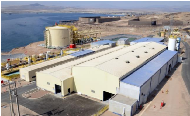
Candelaria desalination facility
