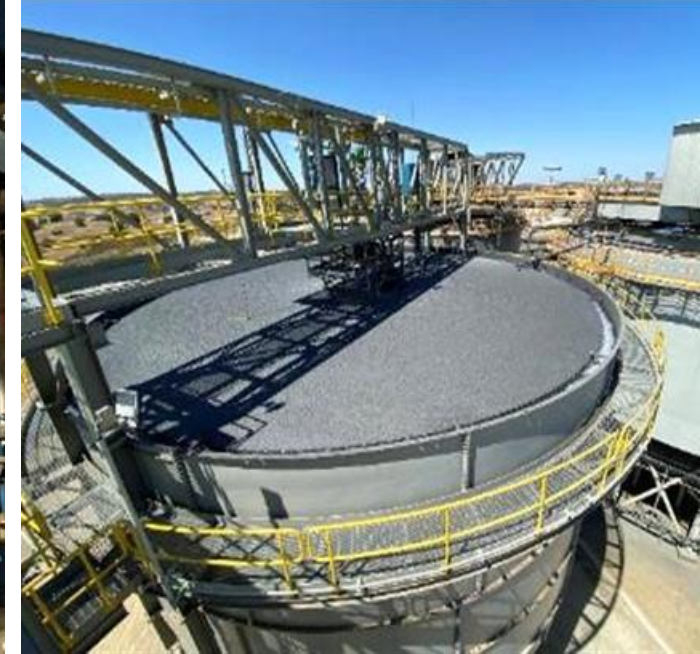
3 rd tailings paste thickener commissioned
