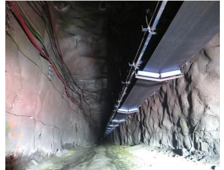
Conveyor Ramp Progress
