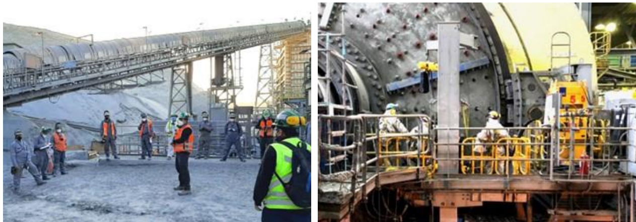
Crusher and mill maintenance – February 2021
