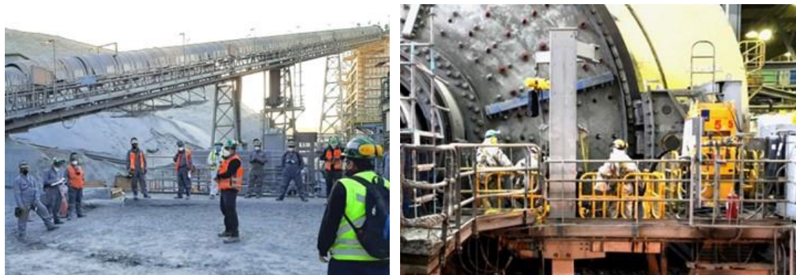
Crusher and mill maintenance – February 2021
