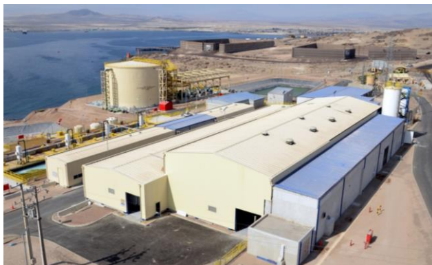
Candelaria desalination facility
