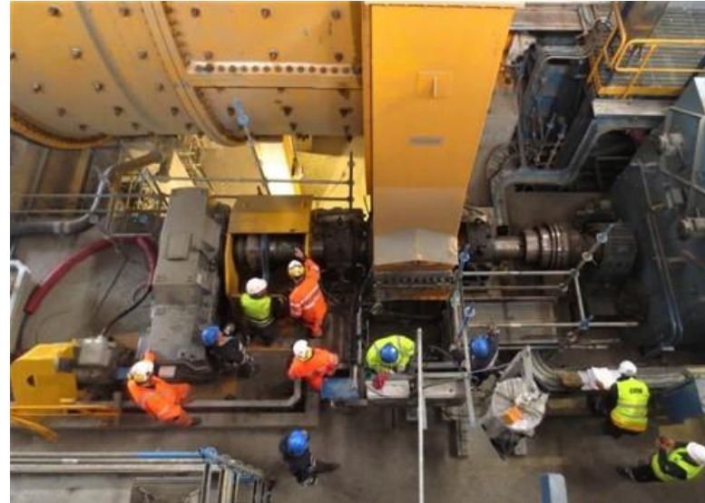
SAG mill commissioning work
