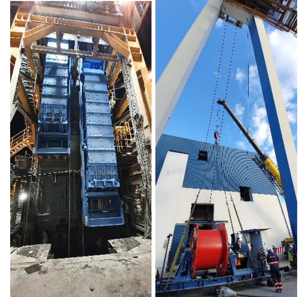
New skips and hoisting rope installed
