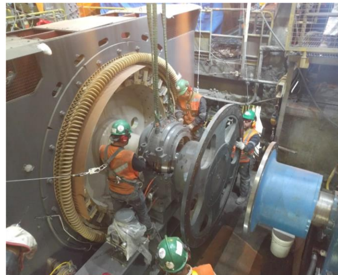
Candelaria Ball Mill 2 motor replacement during Q4/19
