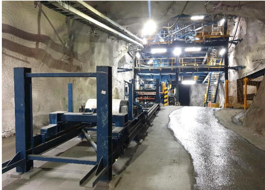
Installation of Transfer Station 3 ongoing
