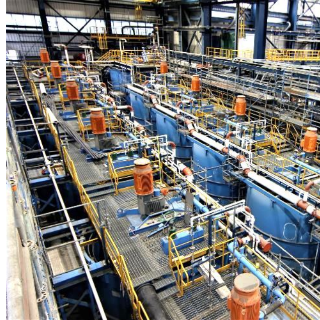
New flotation building piping installation
