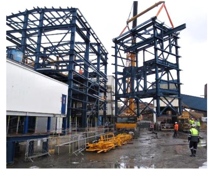
New filtration building and transfer tower steel works
