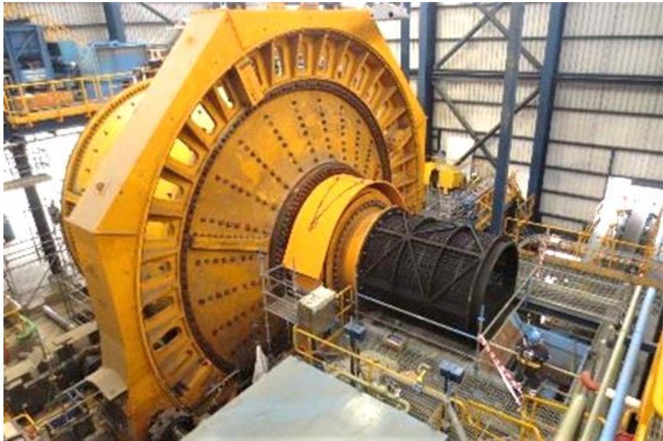
SAG mill motor and hopper installation
