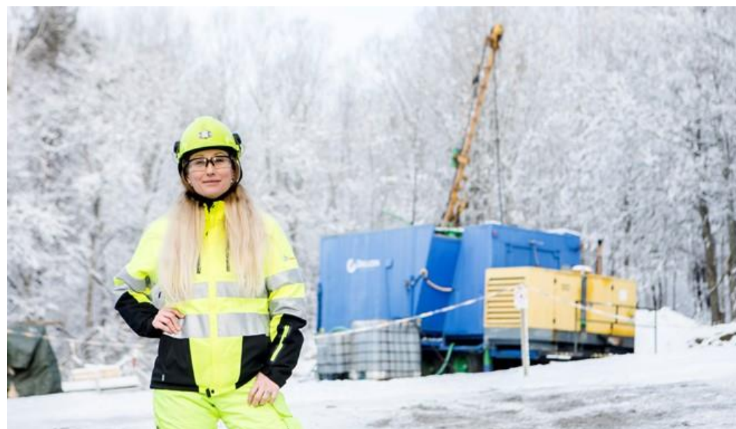
Zinkgruvan – 2019 drilling program
