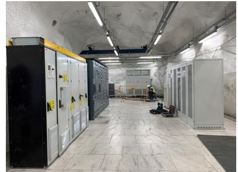
Electrical rooms being installed
