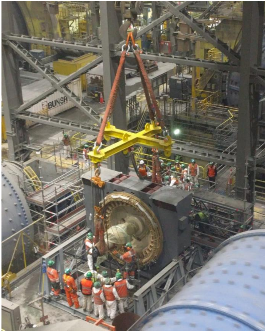
Candelaria Ball Mill 2 motor replacement during Q3/19
