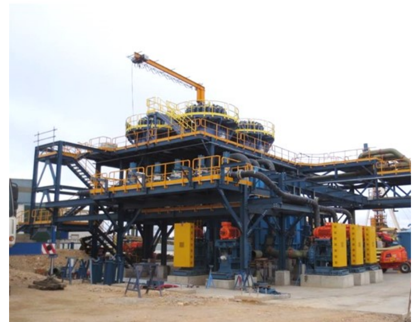
Cyclones area piping installation
