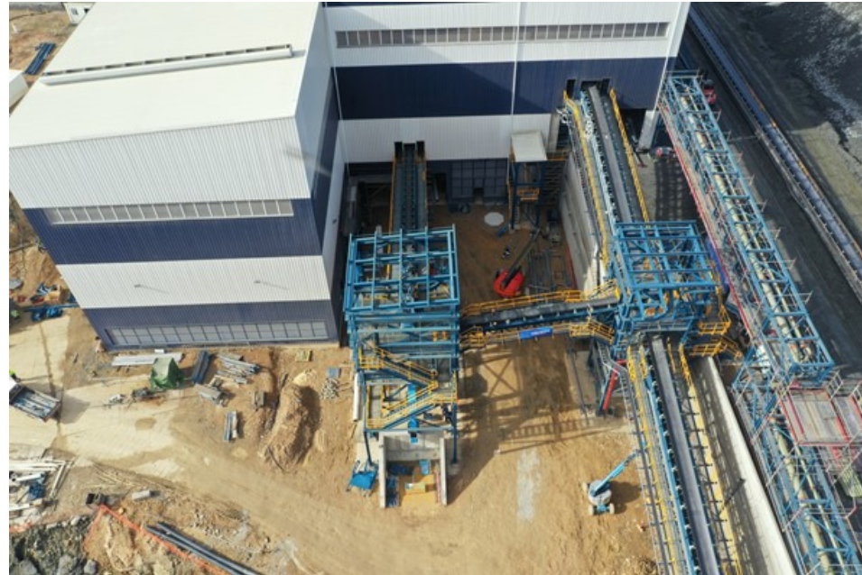
New mill building, conveyors and piping
