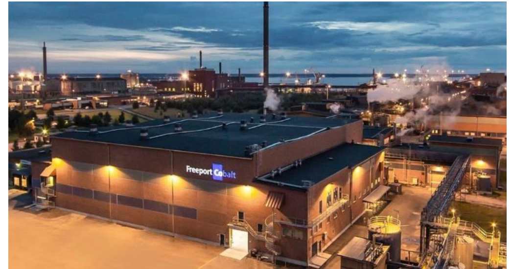
Kokkola Cobalt Refinery
