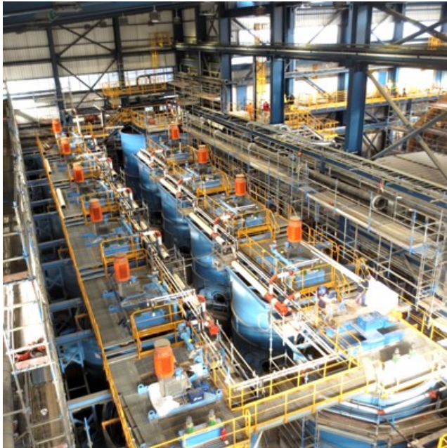
New flotation building piping installation
