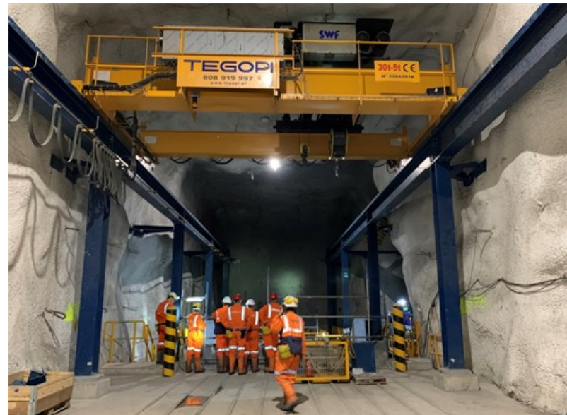
Crusher installed including grizzly and feeder
