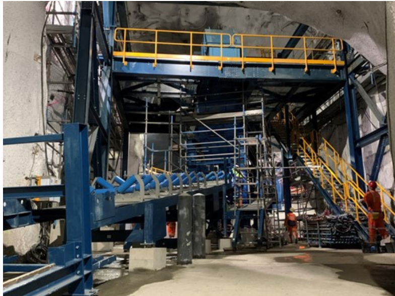
Installation of Transfer Station 2 ongoing
