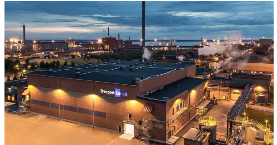
Kokkola Cobalt Refinery
