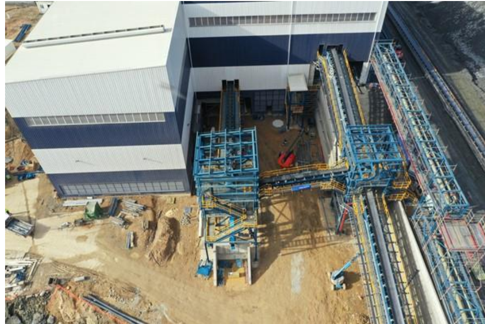
New mill building, conveyors and piping
