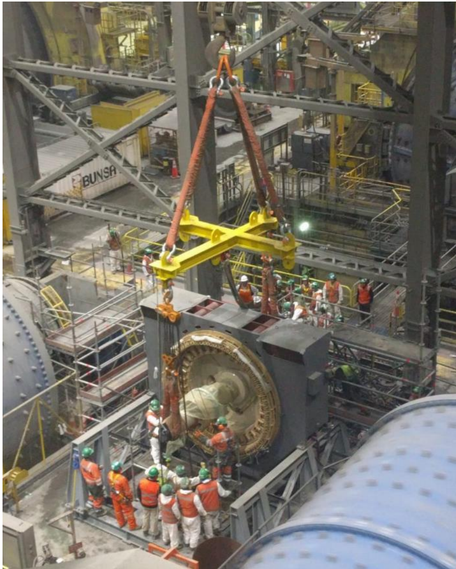
Candelaria Ball Mill 2 motor replacement during Q3/19
