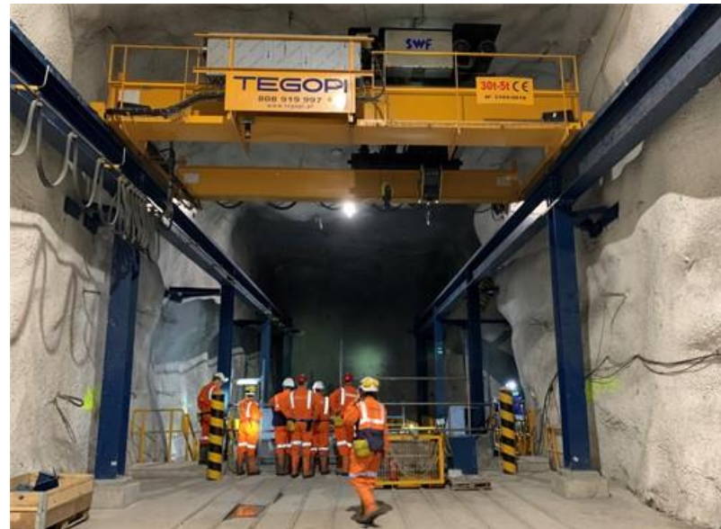
Crusher installed including grizzly and feeder
