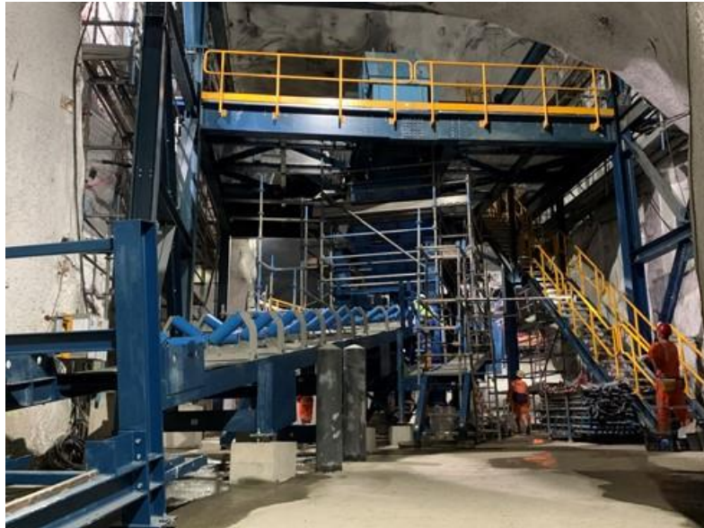
Installation of Transfer Station 2 ongoing
