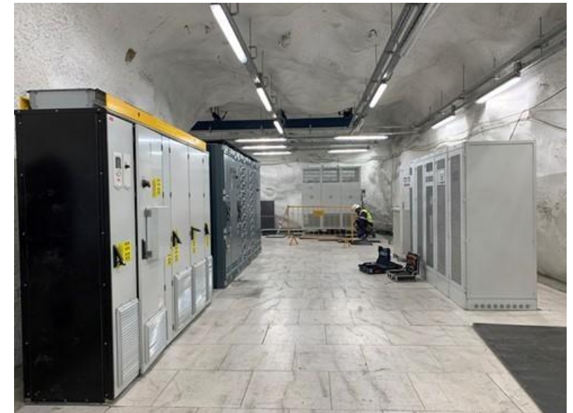
Electrical rooms being installed
