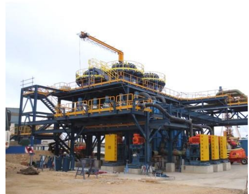
Cyclones area piping installation
