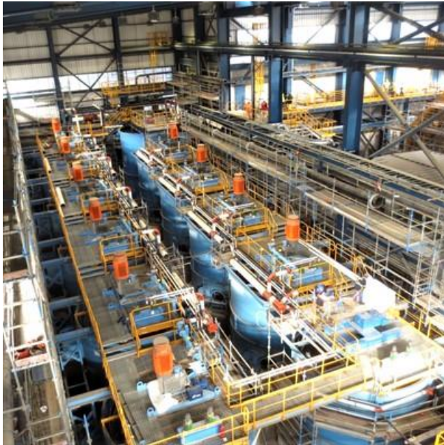
New flotation building piping installation
