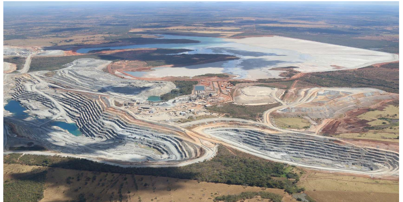
Chapada North and Main open pits in foreground, processing facilities in center, and tailings storage facility in background
