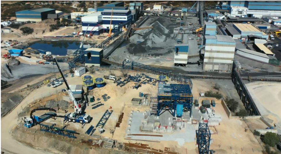
Transfer tower, pipe rack and conveyor construction
