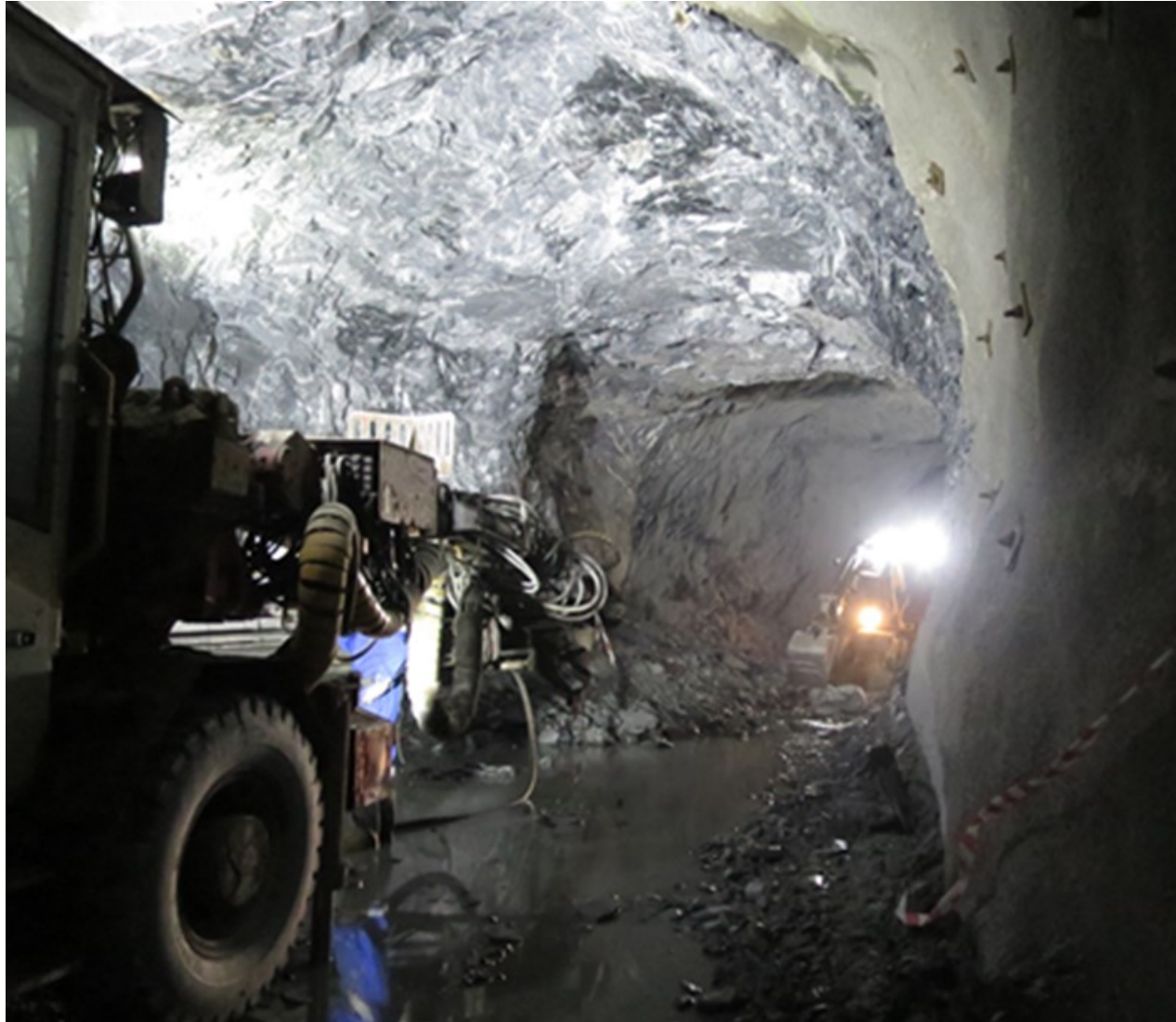
Breakthrough of Ramps 6 and 7
