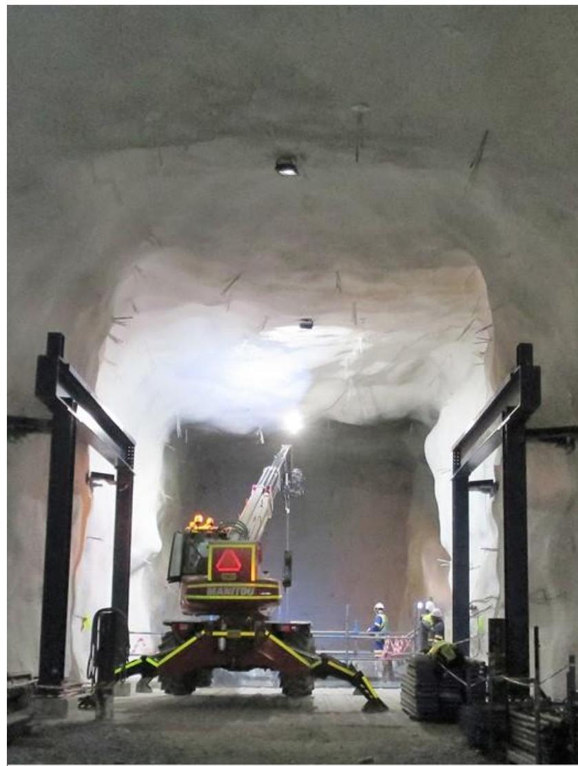
Top of Crusher Chamber
