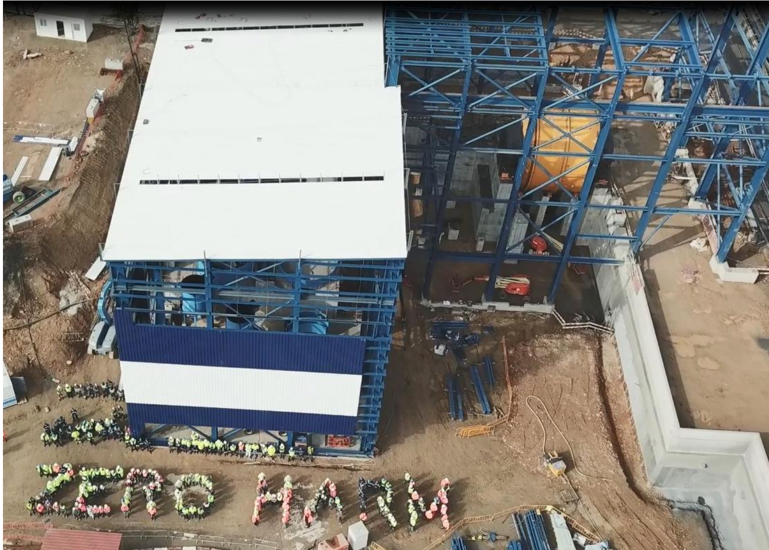
New Zinc Plant Construction – Mid-February 2019
