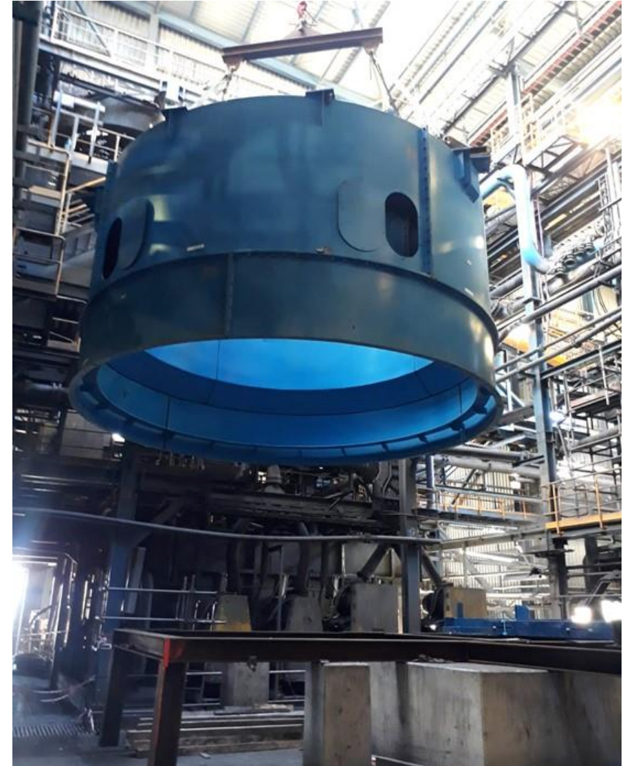
Flotation Cell Installation in Existing Plant
