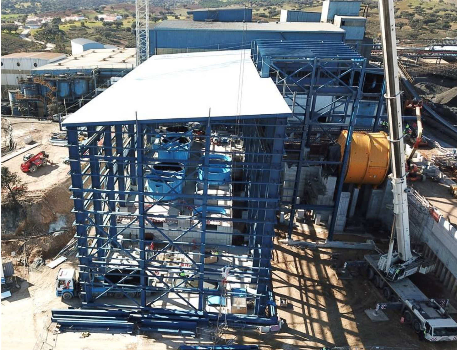
New Zinc Plant Construction – Early February 2019
