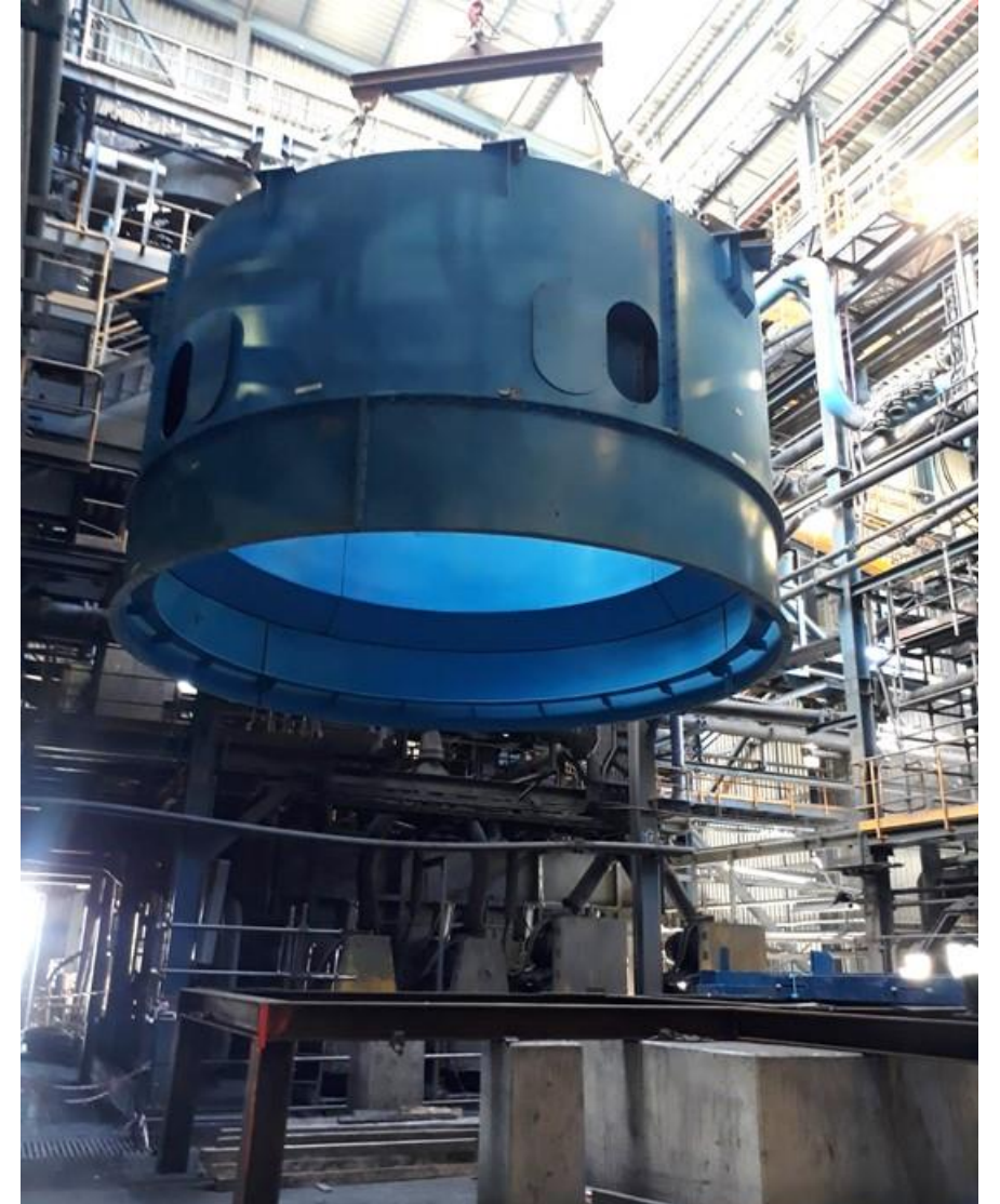
Flotation Cell Installation in Existing Plant
