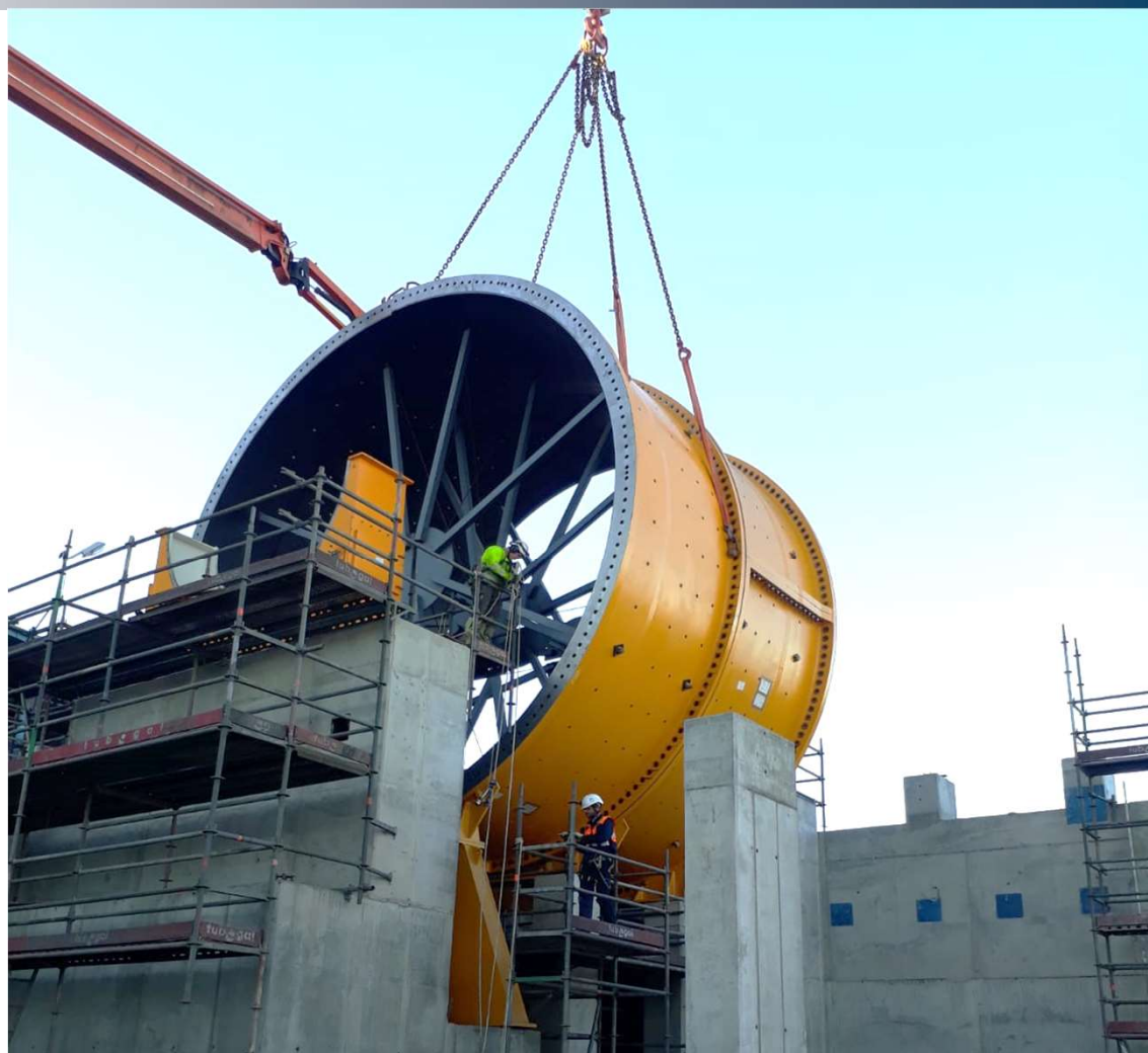
SAG Mill Installation – Mid-January 2019
