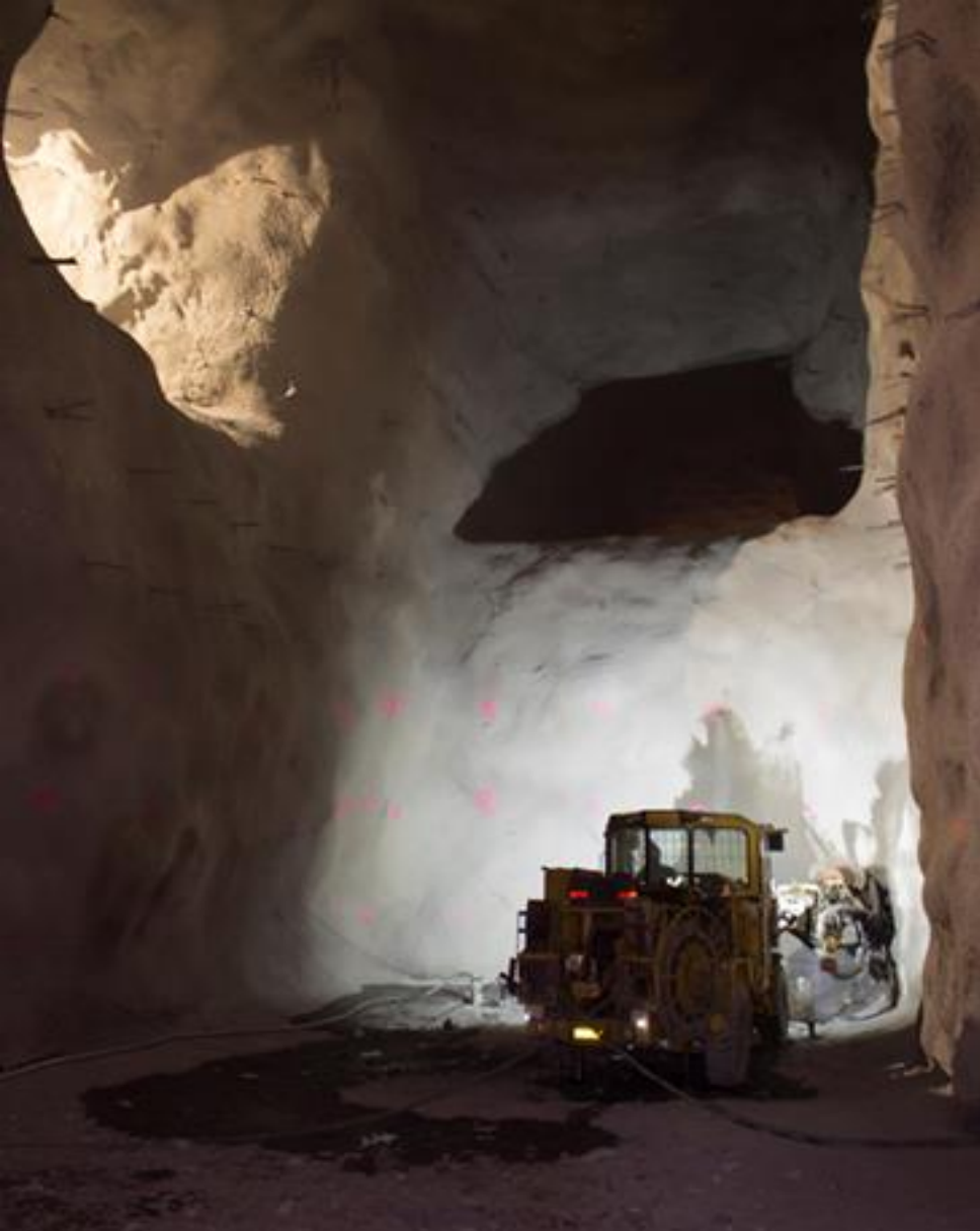
Crusher Chamber Development
