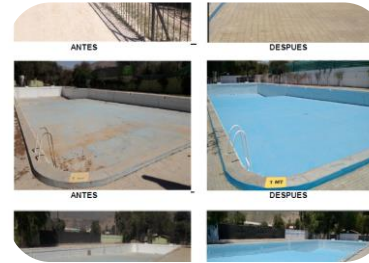
Refurbishment of the Tierra Amarilla Swimming Pool
