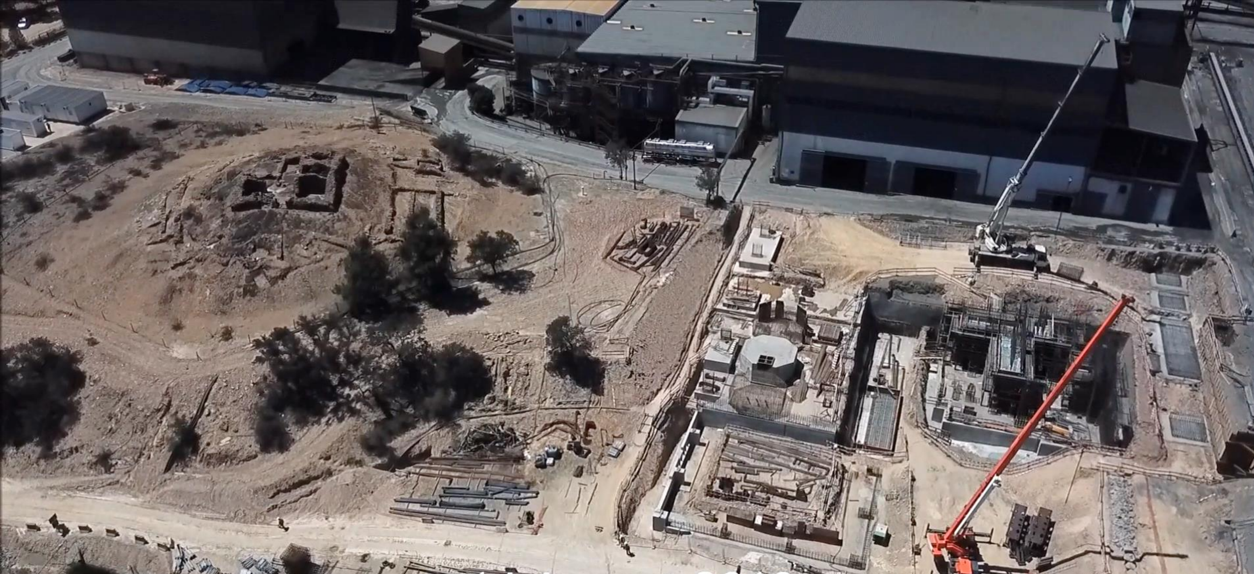
Grinding and Flotation Plant Foundation Surface Construction – August 2018
