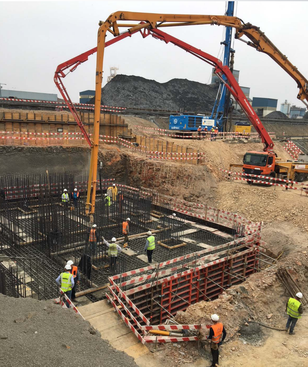
Pouring of Mill Foundation
