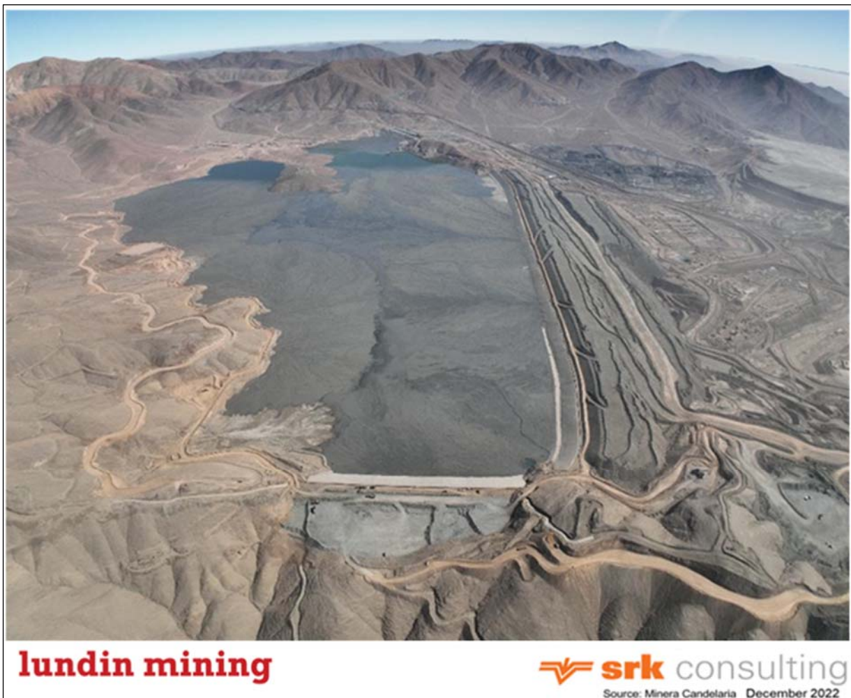
Figure 54: Los Diques Tailings Storage Facility, August 2022 (Looking North-West)
