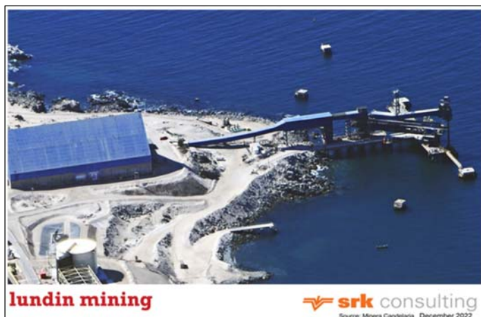
Figure 52: Aerial view of the Punta Padrones Port Facility
